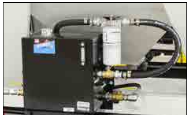
Fig 9 - Hydraulic oil reservoir and filter
